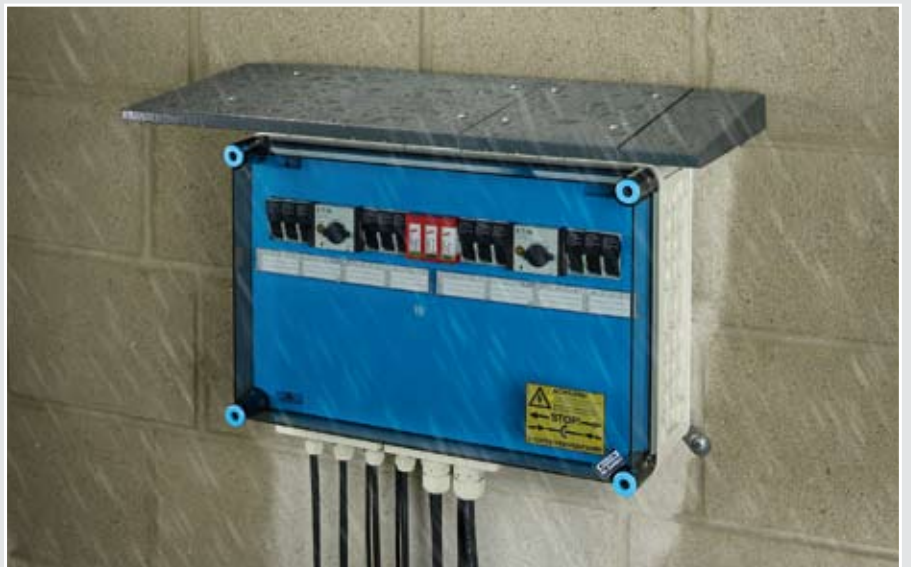
Example: Mi distributor protected by canopy
